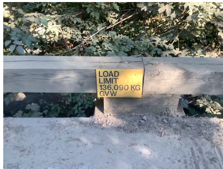
Load Rating Sign
