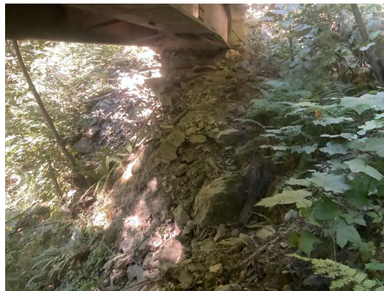
Right Bank Abutment when facing downstream
