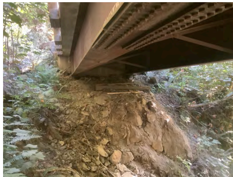
Left Bank Abutment when facing downstream
